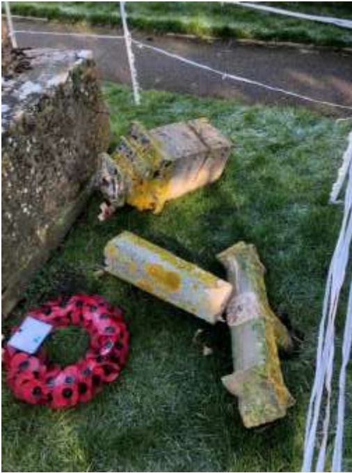
Broken sections on the ground
